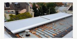
The Albatross Conservatory Awning system is constructed to secure the fabric on the top roller and front rail only. While the sides of the fabrics still run via track channels with roller guides, the awnings can not be used during heavy rains and strong winds.
