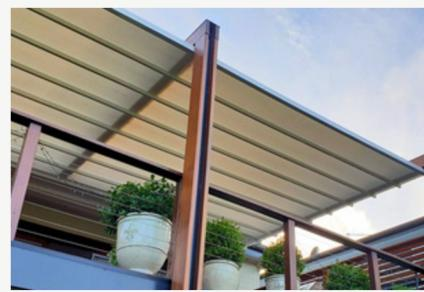
Self-supporting system constructed with natural timber support frame.
